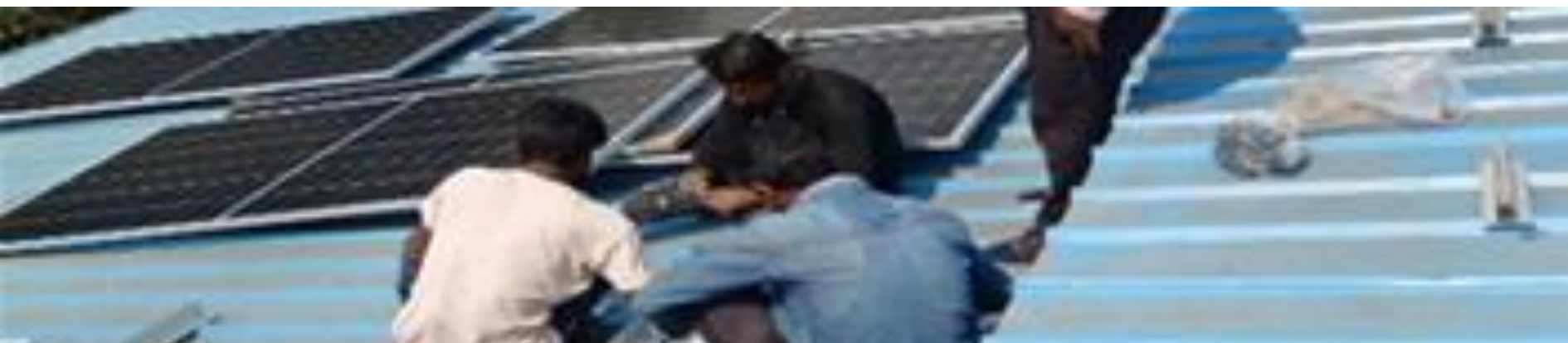
Solar panels are installed on the Solid Waste Management shed rooftop in Karad Municipal Council.
