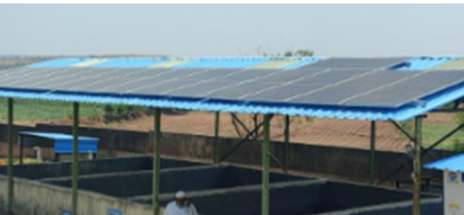
SDB shed and solar panels installed at Vita FSTP.
